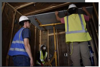
During Week 5 of construction, BUILD members suited up in protective gear to complete the insulation. With that finished, they began installing the ceiling and wall panels they had prepared in previous weeks. As each panel went up, the clinics truly began to take shape.
